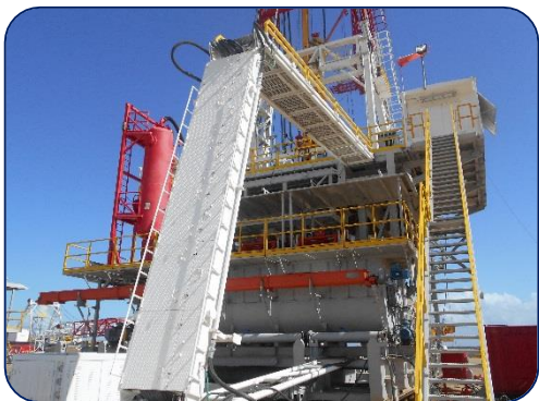
Substructure – Front View
