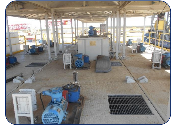
Mud Pit Room
