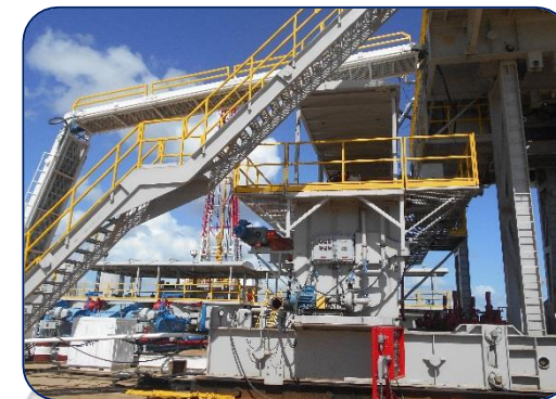
Substructure – Lateral View
