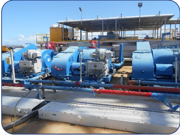
Triplex Mud Pumps
