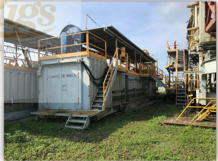
MUD TANK SECOND
