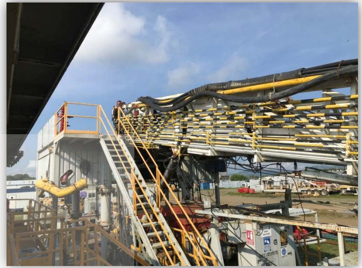
MAST AND SUBSTRUCTURE
