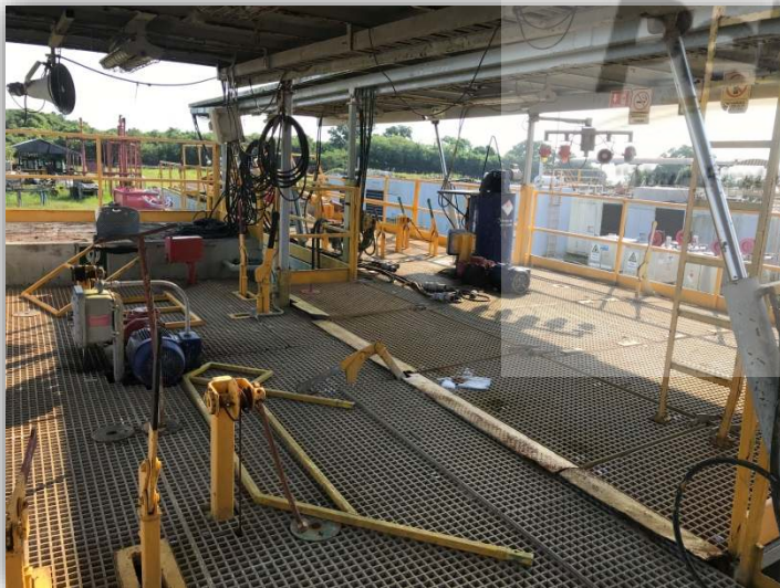
MUD TANK SECOND
