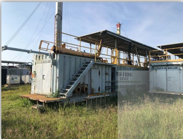
SUCTION MUD TANK
