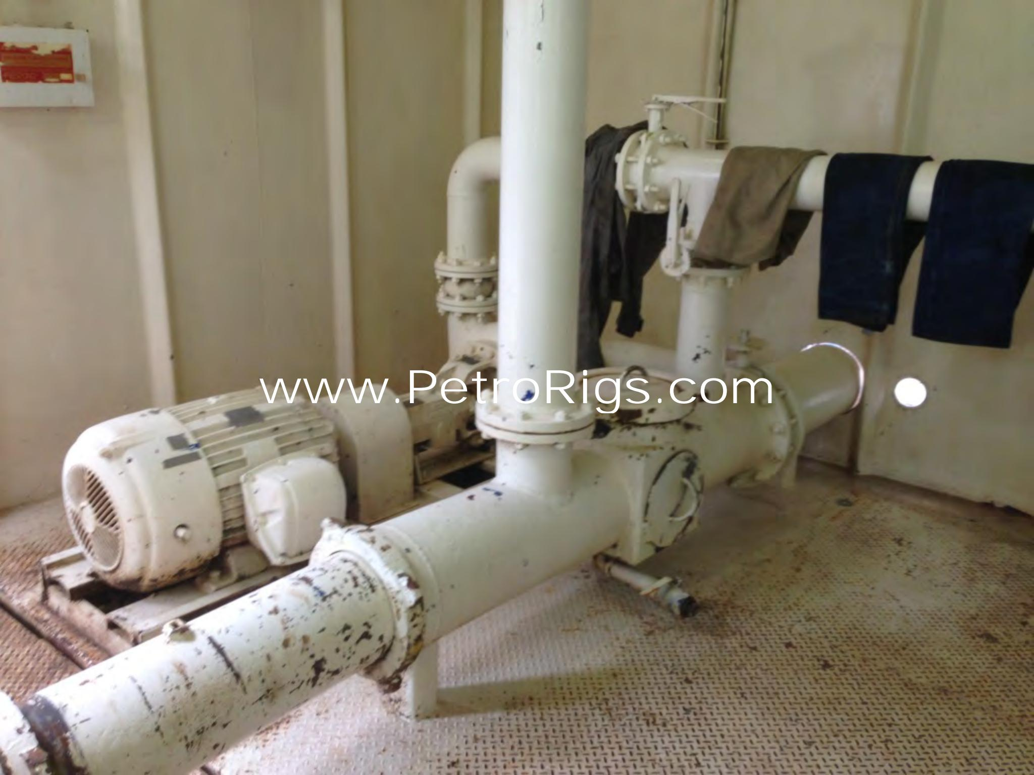
A photograph of an industrial pump unit. On the left, a white electric motor with a fan is mounted on a metal base. A large, light-colored pipe with dark spots runs horizontally across the frame, connected to the motor and a vertical pipe. The vertical pipe leads up to a white pump body with a valve. Several dark towels or cloths are draped over the top of the pump. The background shows a plain wall and a small red sign in the upper left corner.
