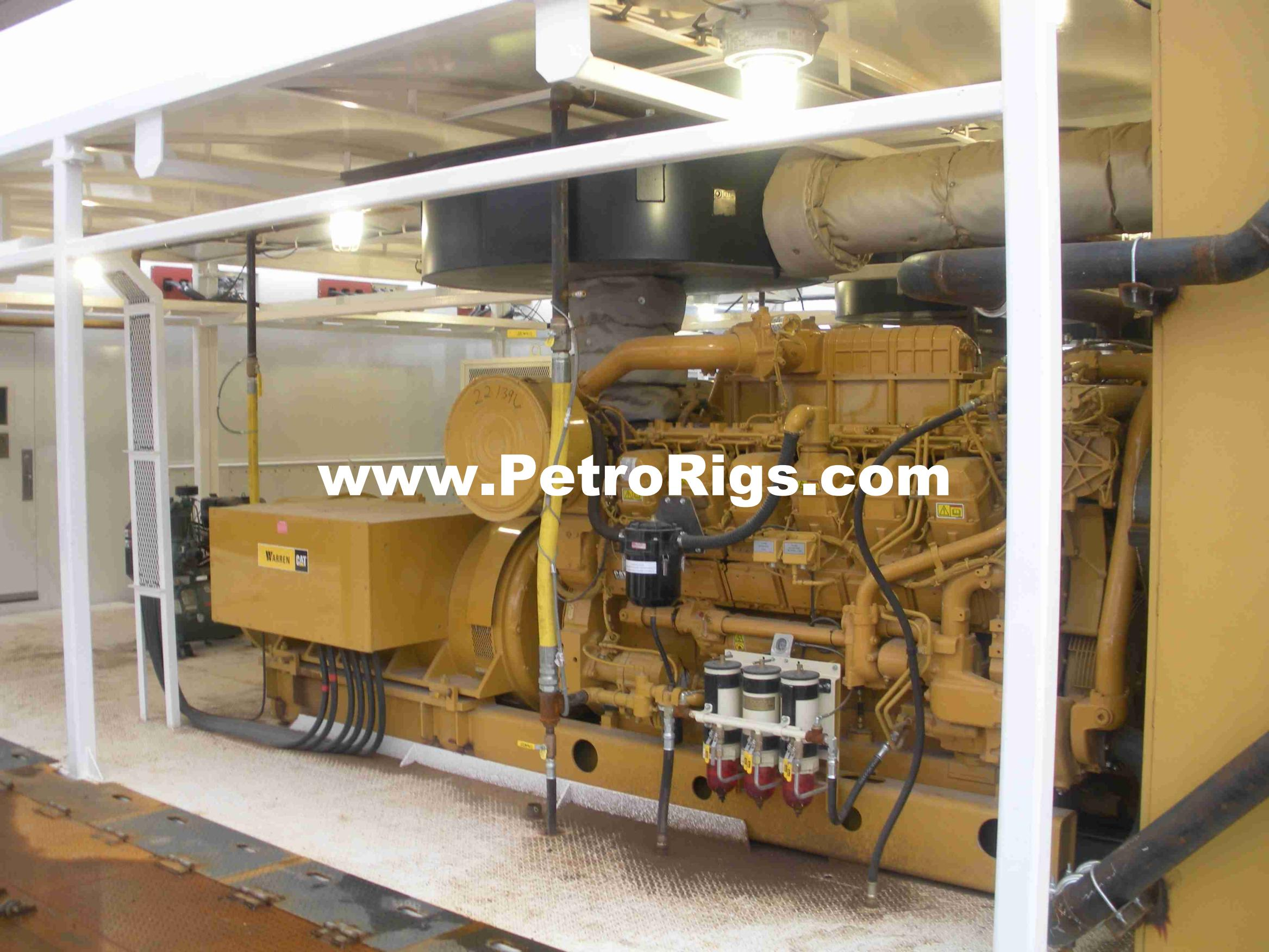
A large yellow Caterpillar generator set is shown in an industrial setting. The generator is mounted on a metal frame and has various pipes, hoses, and electrical components attached. The number "221396" is visible on a component near the engine. The background shows a white metal structure and some equipment.
